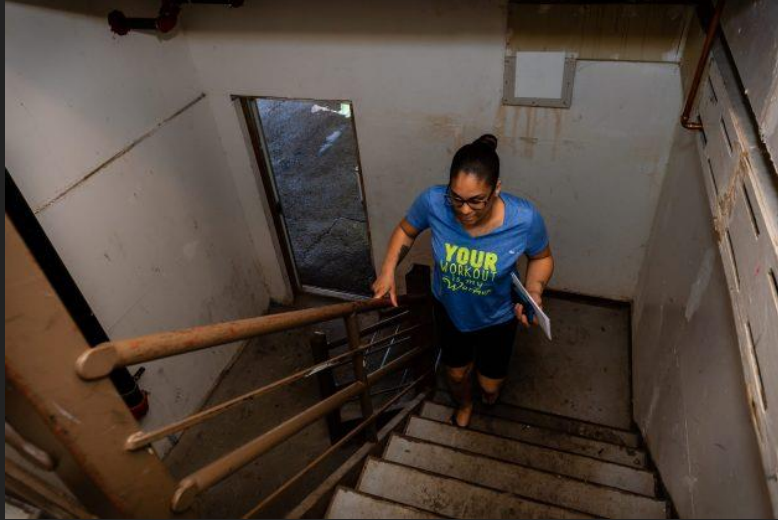
Yashira Santiago, a tenant at the Pine Hill Towers uses the stairs to walk up to her apartment on Friday. Yashira was using the stairs since the elevator wasn't working when she tried to use it. The elevator recently has not been working forcing tenants to use the stairs. Bill Shettle Republican-American
