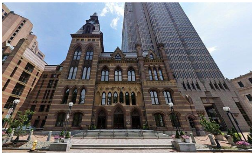
New Haven City Hall. Photo: Google
